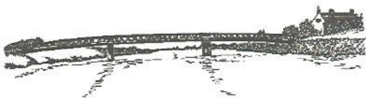
The old timber Magdalene Bridge was replaced in 1913 by the existing steel lattice girder bridge. (Centre span 84 ft). It is due to be reconstructed in the near future.
